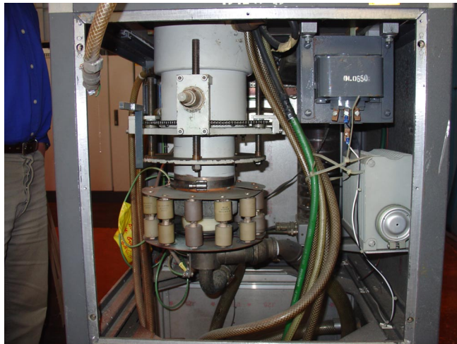
Inspection at Daresbury
